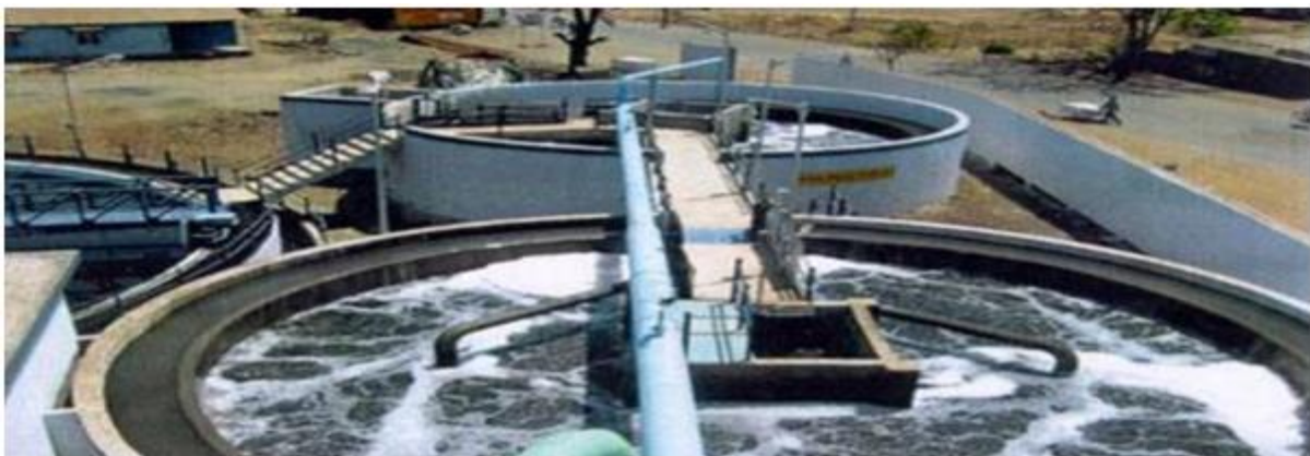
Figure No 35. Aeration Tank
